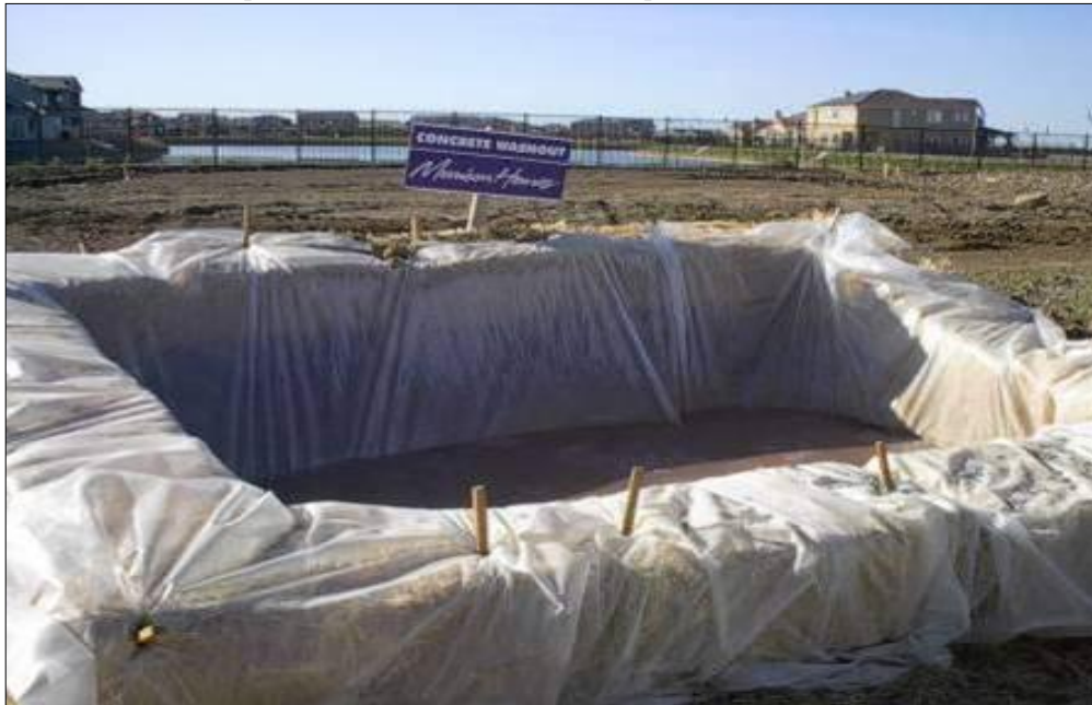
Plate 5-1 Concrete washout area
