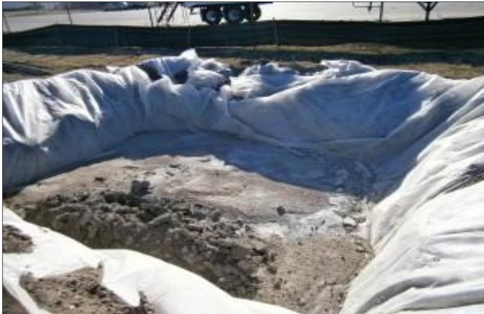
Plate 5-2 Concrete Wash Out Area
